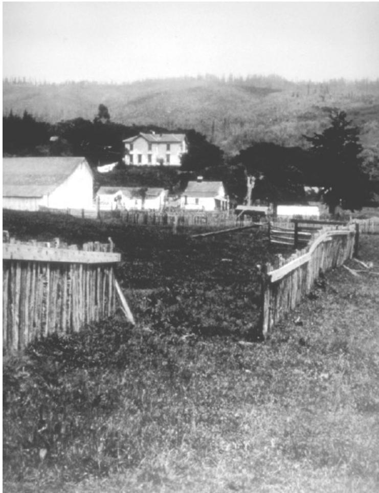
1906 San Francisco earthquake
